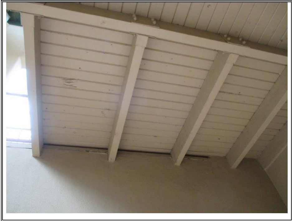
WOOD DECKING -REC BUILDING (TYPICAL)
