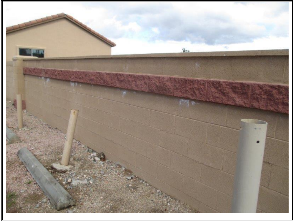
CONCRETE BLOCK WALLS (TYPICAL)
