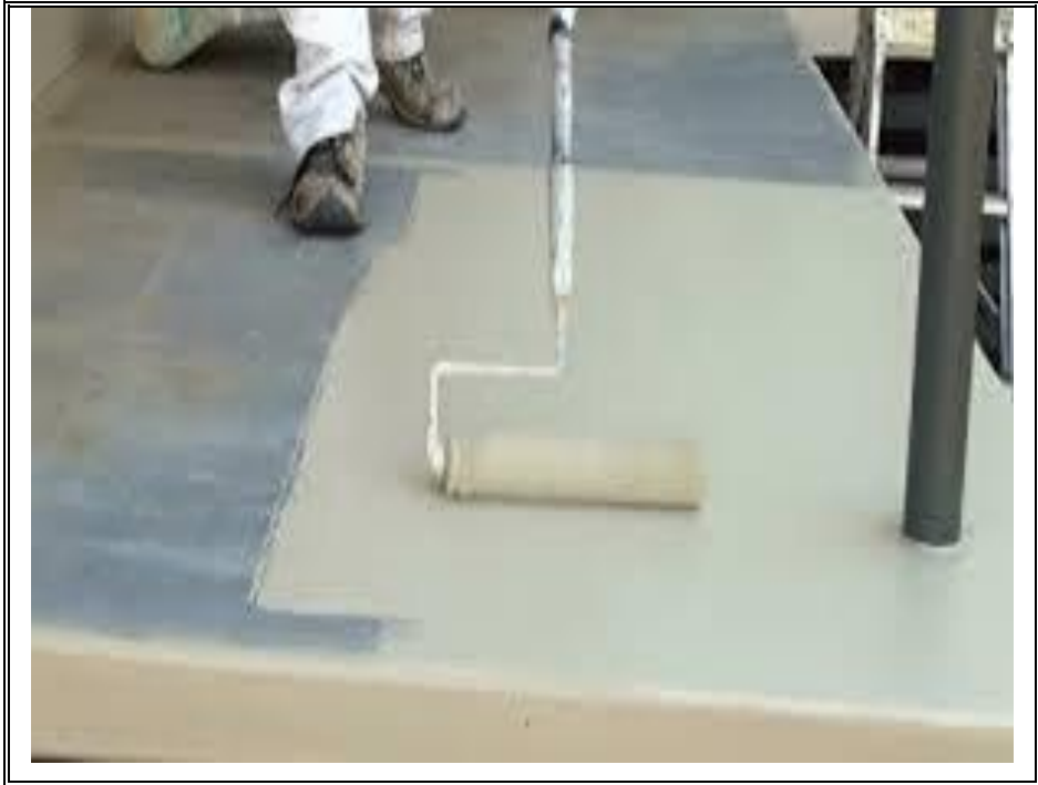
MEMBRANE DECKS-COATING (TYPICAL)
