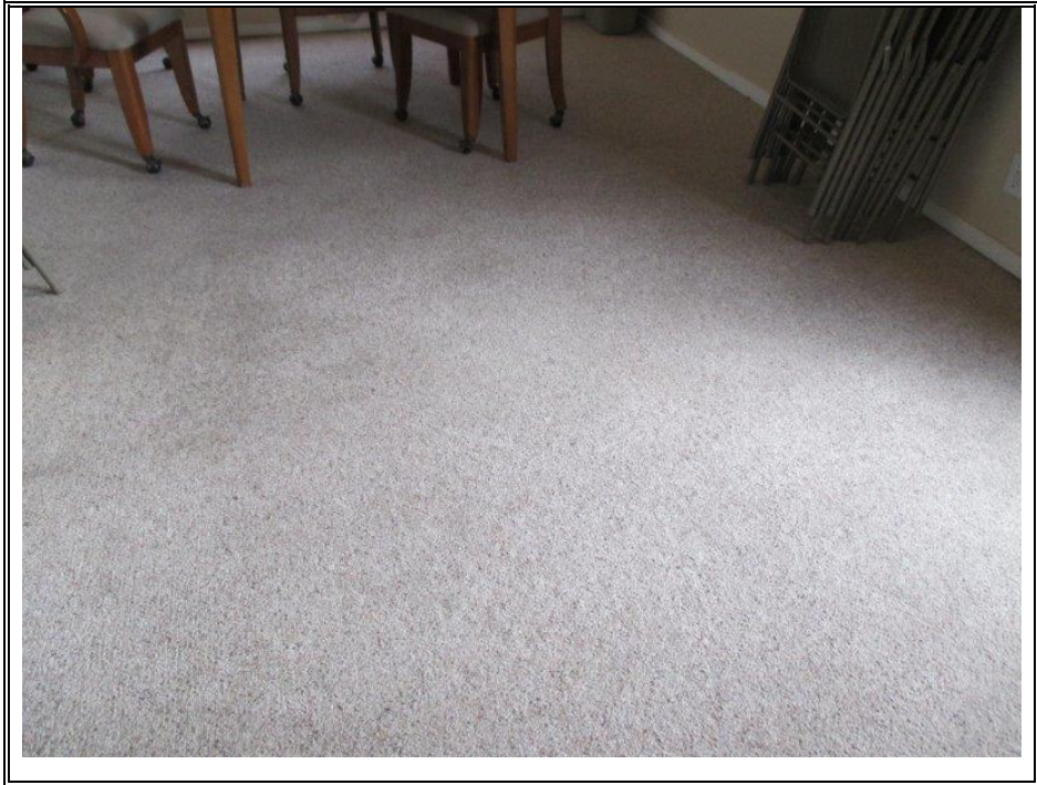
CARPETING- REC BUILDING (TYPICAL)
