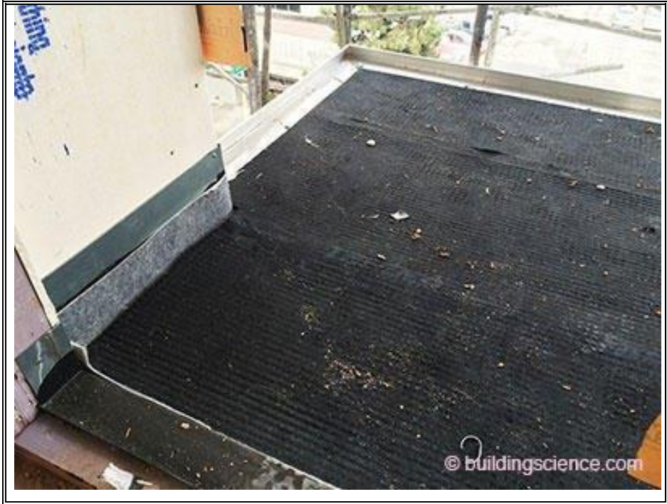
MEMBRANE DECKS-RESURFACE (TYPICAL)
