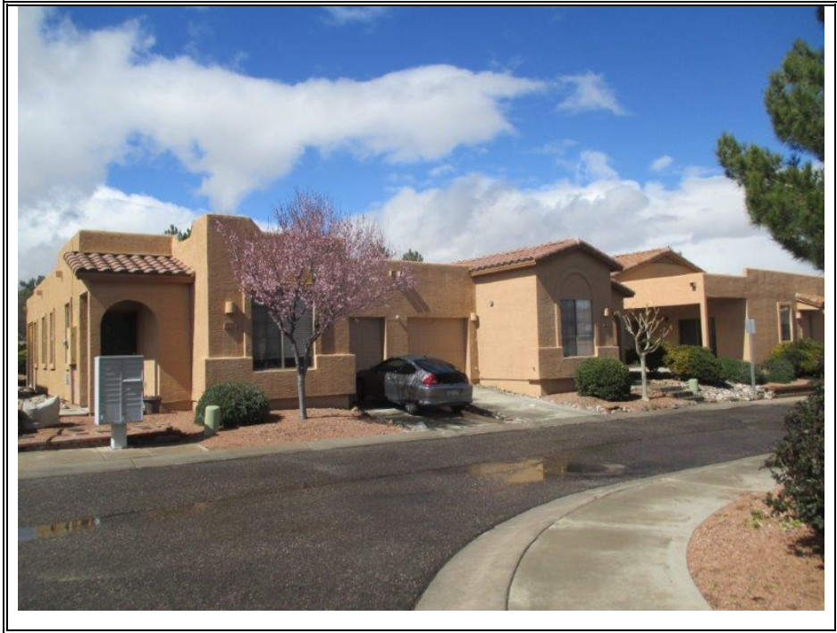
FOUNDATIONS/STRUCTURAL FRAME--REC BUILDING (TYPICAL)
