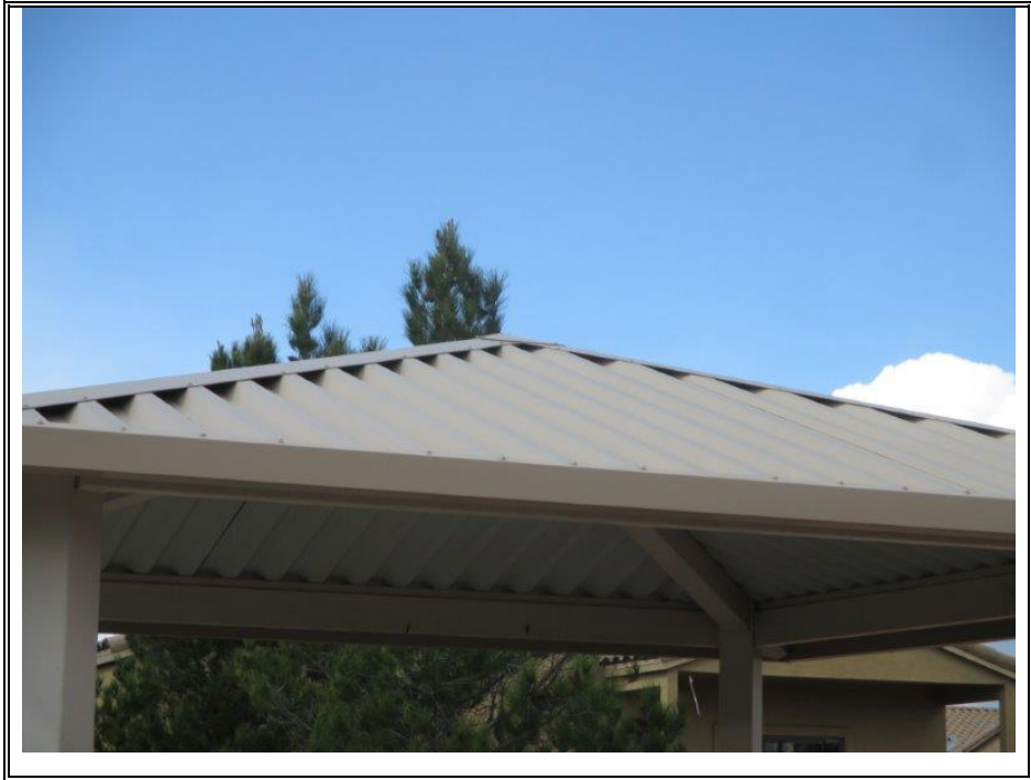
STANDING SEAM ROOF -REC BUILDING (TYPICAL)
