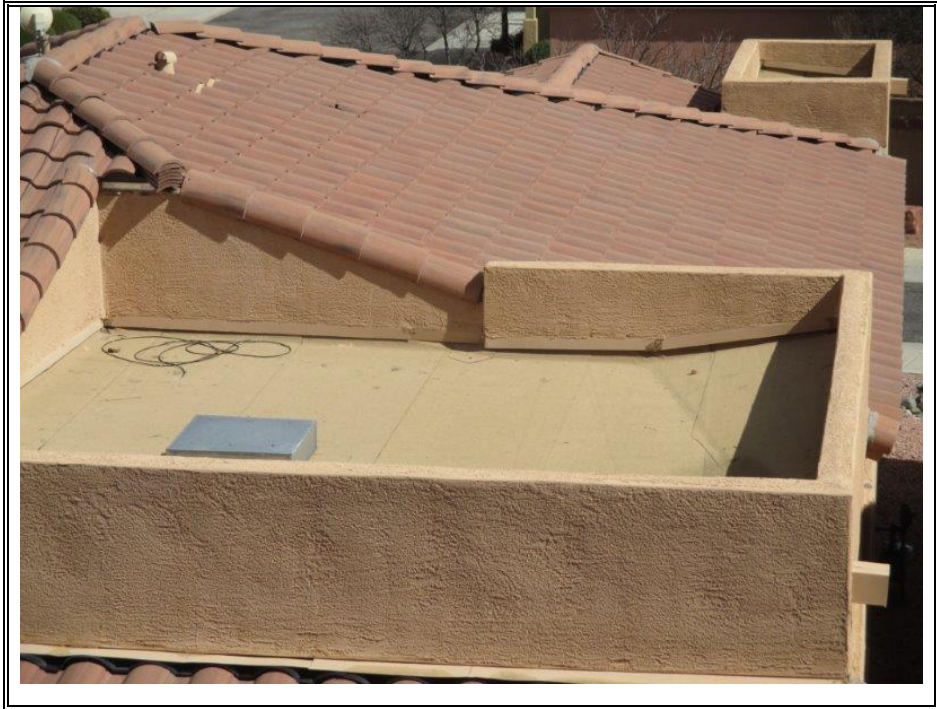
CAP SHEET ROOF – REC BUILDING (TYPICAL)
